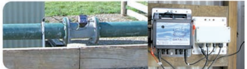
Irrigation Watermeter Installation
